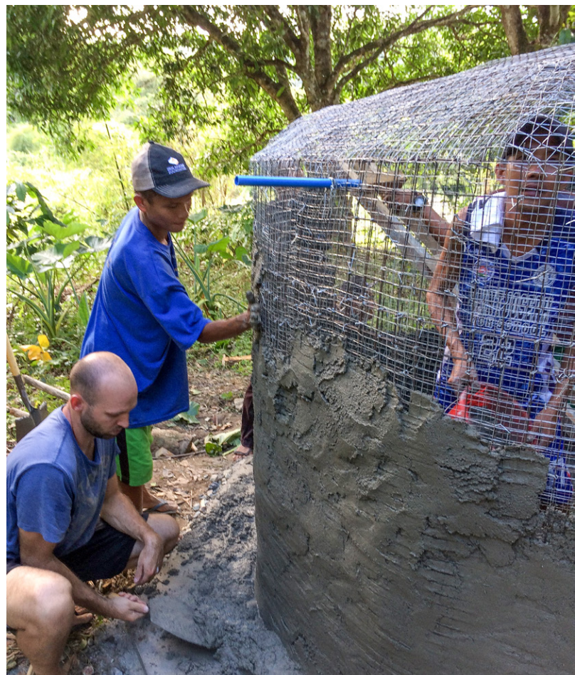
Building the water tank. photo by Alex Williams
